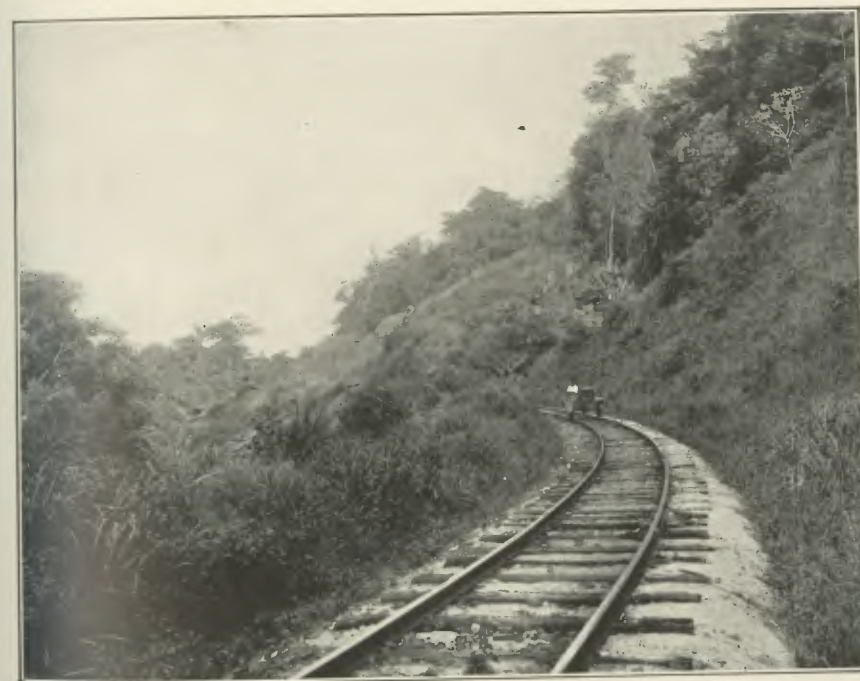
ON THE BLACKALL RANGE, NORTH COAST RAILWAY
